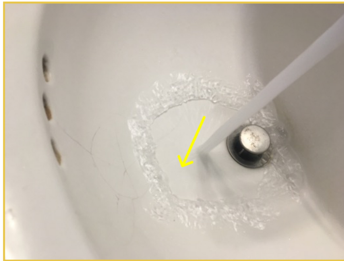
Cracked Main Floor Hall Bathroom Sink
