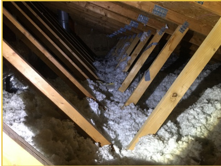
Attic With Fiberglass Insulation
