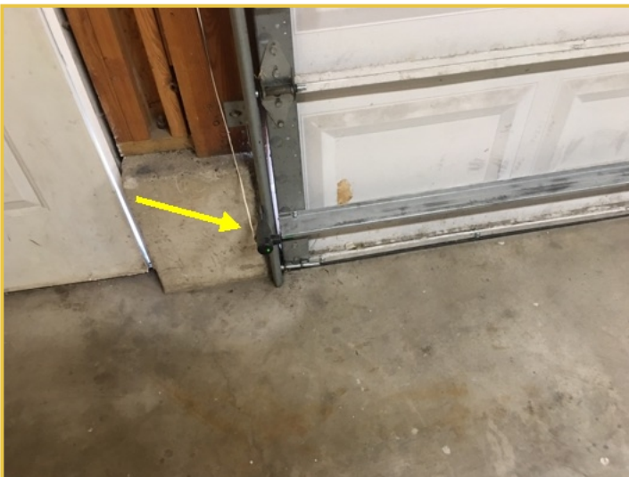
Garage Door Reverse Sensors Too High
