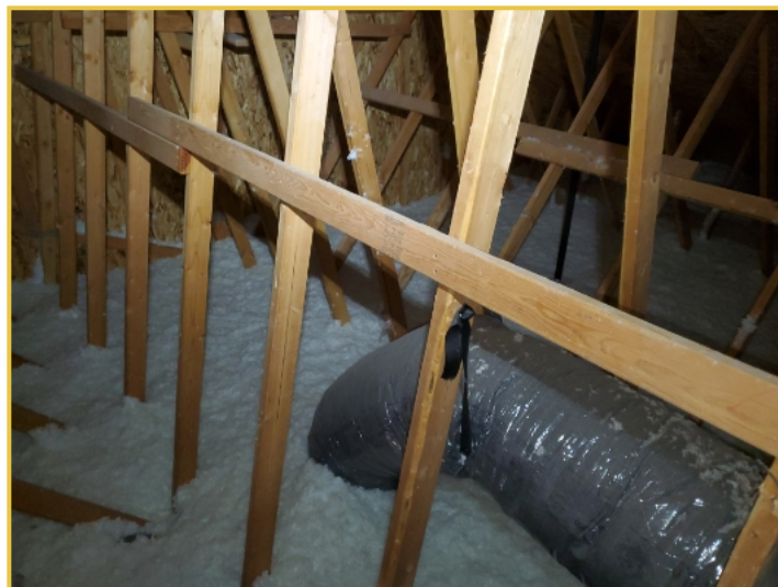
Attic With Fiberglass Insulation
