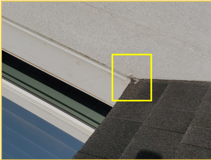
Short Kickout Flashing
